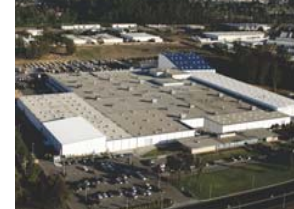
Santa Maria, CA - Manufacturing Plant
