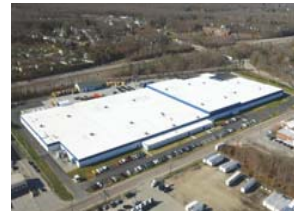
Cumberland, RI - Manufacturing Plant
