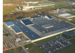
Richmond, KY - Manufacturing Plant
