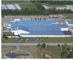
Orangeburg, SC - Manufacturing Plant
