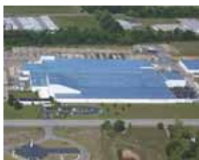
Orangeburg, SC - Manufacturing Plant
