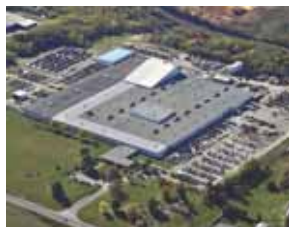
Richmond, KY - Manufacturing Plant
