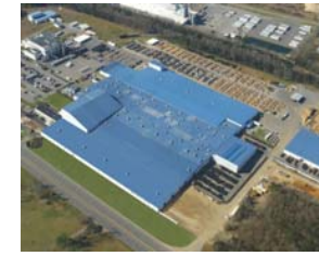
Orangeburg, SC - Manufacturing Plant
