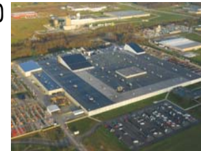
Richmond, KY - Manufacturing Plant
