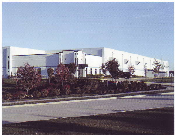
Pittsburgh Service Center 120 Solar Drive Imperial, PA 15126 (724) 899-4300 FAX:(724) 899-4320
