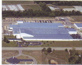
Orangeburg, SC - Manufacturing Plant
